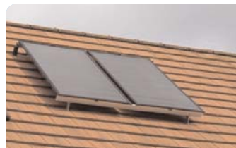
4m 2 of flat plate collectors (Energy Saving Trust)
